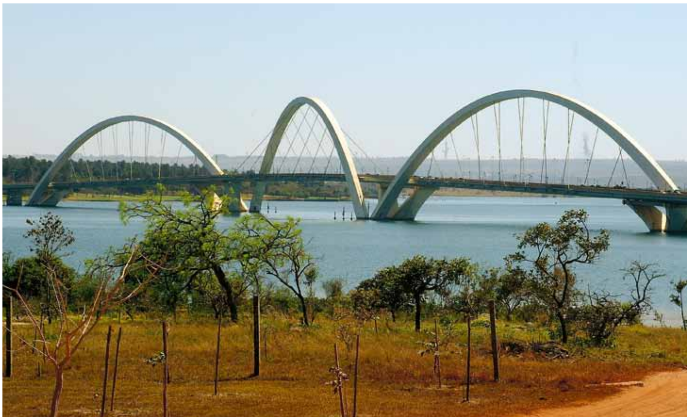
J.K Bridge Foto: Emelie Andersson.
